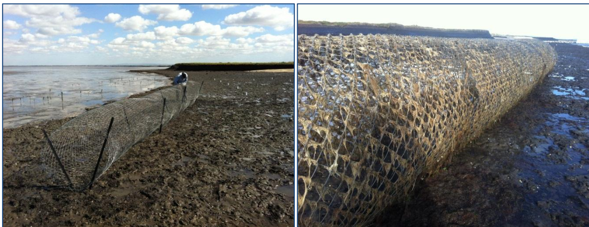
Figure 34: Enviro roll when constructed (left) and 4 months after construction (right) showing significant build-up of algae and other debris.
