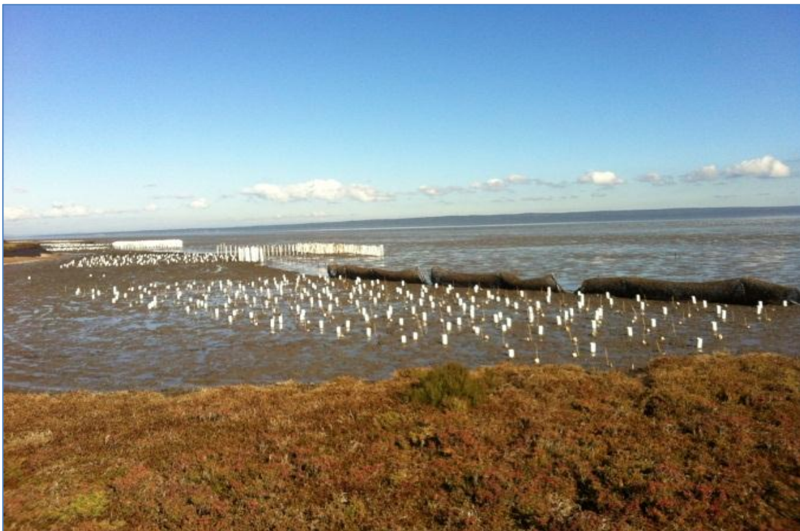
Figure 36: Experimental site viewed from north end. Enviro rolls in the foreground with two pile fields visible (one under construction) in the background. Planting plots with PVC pipe tree guards visible in lee of structures.
